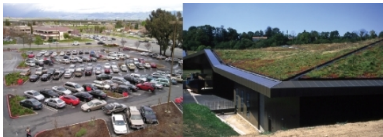
Figure 18.30: Impervious surfaces (left) fragment habitats, increase runoff, degrade water sources, reduce photosynthesis, and effectively increase CO in the atmosphere. In the U.S., they cover an area of land almost the size of Ohio. Permeable pavements and green roofs (right) are beginning to reverse their effects.
